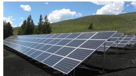
Solar energy is a prime example of renewable energy.
