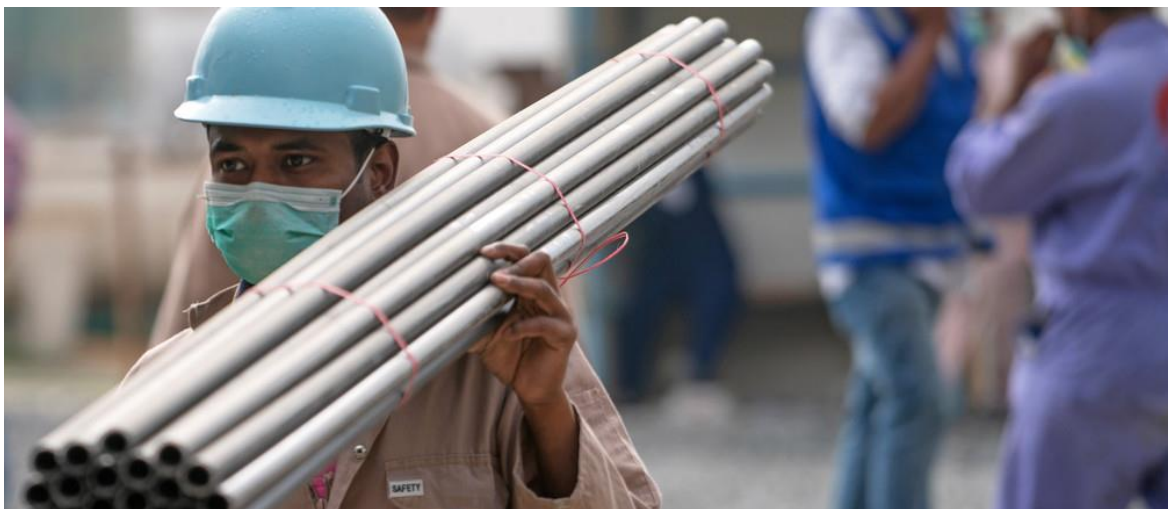
A Worker in the Scene of Infrastructure Restoration
