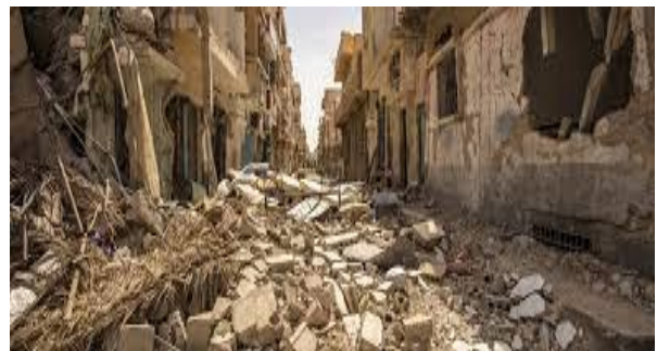
Poor Living Condition in Syria
